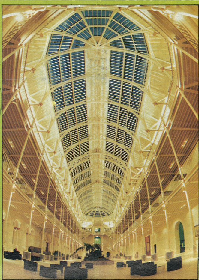
The main hall of the Royal Museum of Scotland in Edinburgh has been relit using Thorn Lighting's Arcstream metal-halide lamps. Single-ended 150W lamps in specially-designed quarter-sphere uplights were used. Low-voltage tungsten-halogen lighting from the Lightstream range provides spotlighting. Electrical load has sunk to 16.8kW from a previous 20.4kW fluorescent/PAR 38 scheme. Thorn Lighting 01-363 5353.
