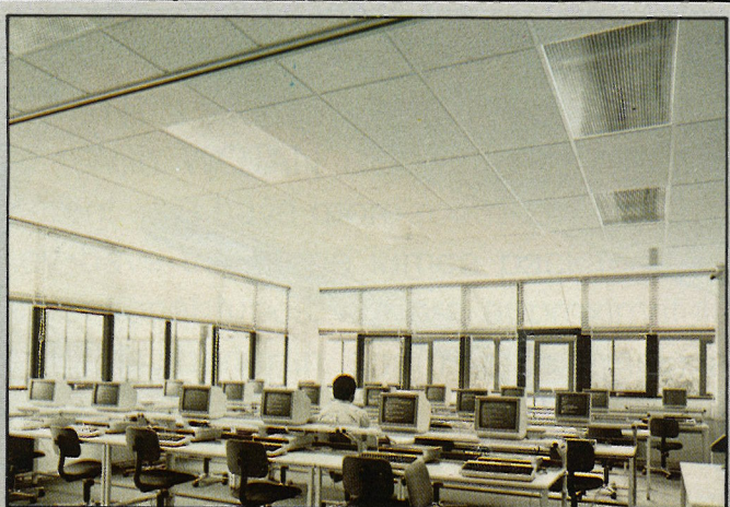
The new, purpose-built, Cripps computing centre at the University of Nottingham is lit using Tamplate low-glare modular luminaires. Tamplate design engineers arranged the luminaires to suit the known layout of the work stations. The main object was to avoid reflections in VDUs. The final design is said to satisfy CIBSE technical memorandum 6, Lighting for visual display units. Details from R Lacey 0952-586818.
